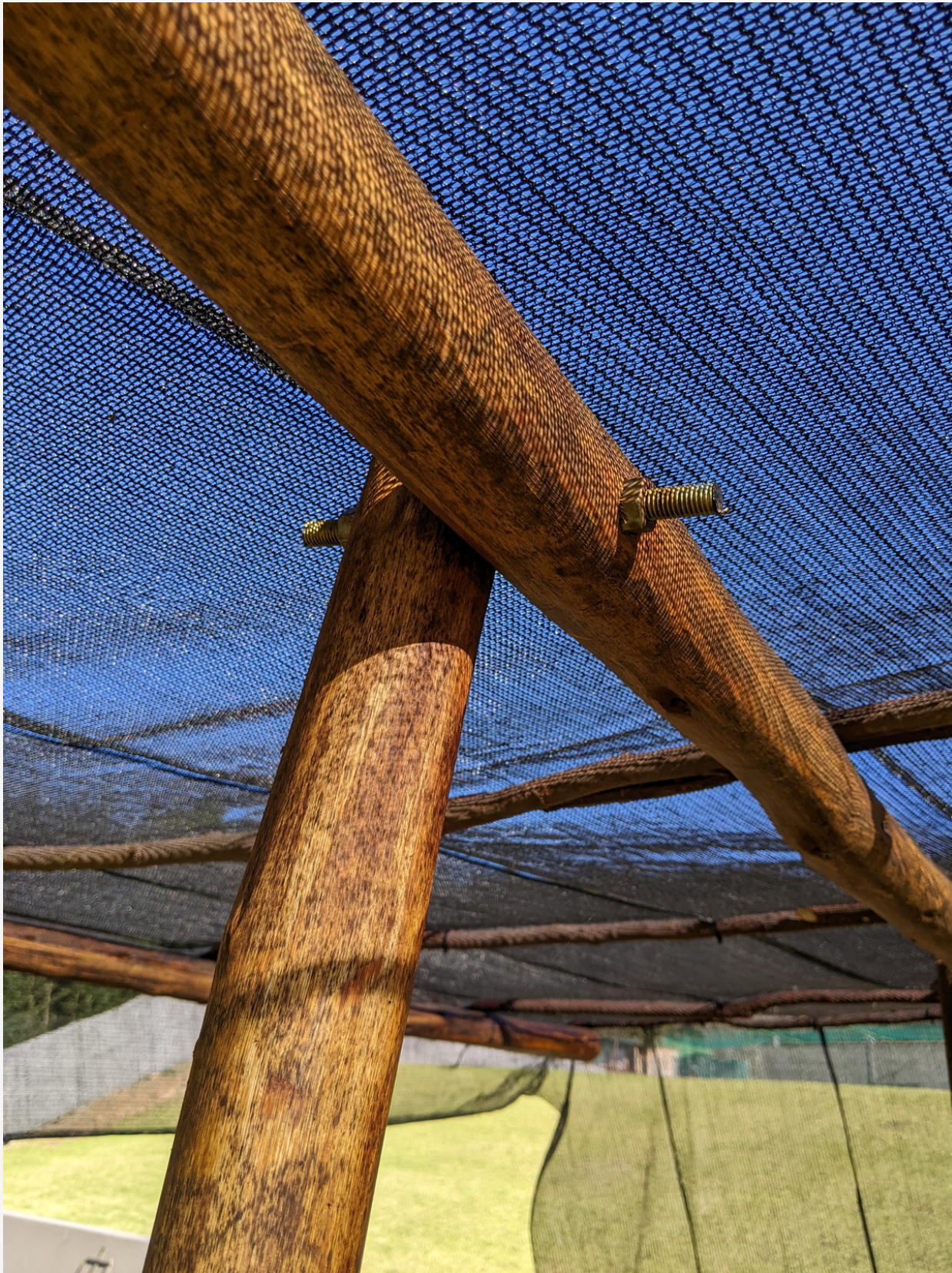
Visual of threaded rods with nuts fastened to secure gum poles
